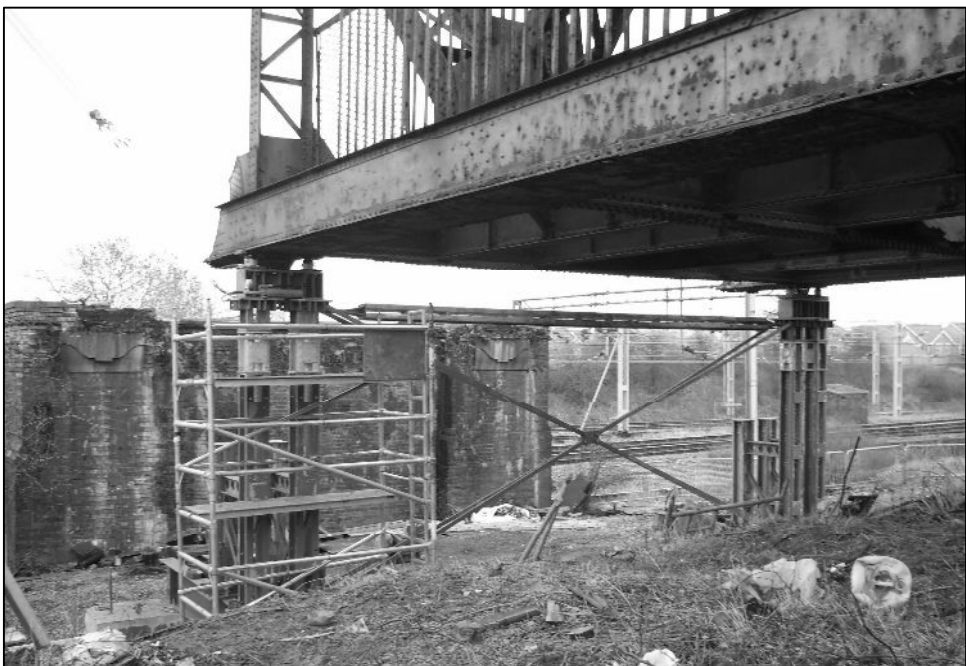
26 th Dec - The remaining section on the south side is supported on jacks.
