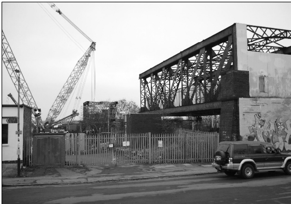
25 Dec : After removal of the main section the two remaining parts of the bridge on both sides of the tracks can be seen in this view from the south end of the structure. photo : David Boulton
