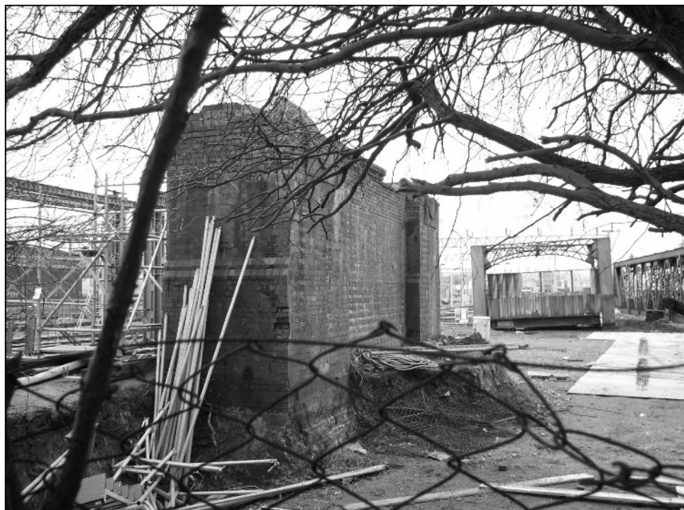
5 Jan. - The bridge support at the north side of the tracks after the remaining north section has been lifted and grounded nearby. The large section lifted on 25 Dec. can be seen alongside to the right. photo: David Boulton
