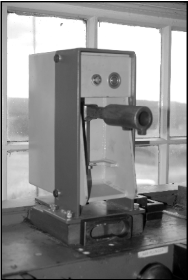
Below: The new Annett's key machine at Thoresby Colliery Jnct. signal box.
