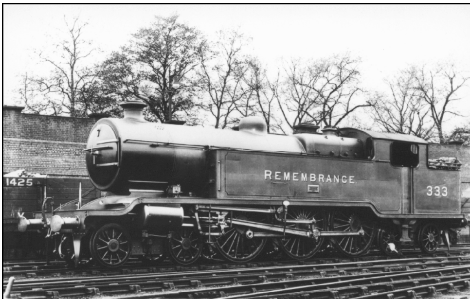
Lawson Billinton's Baltic tank for the LB&SC no.333, the most magnificent of a splendid type. In 'Brighton' days the war memorial status of 'Remembrance' was emphasised by a sombre battleship grey livery: the Southern later enhanced her grandeur with a coat of green and nameplates.
