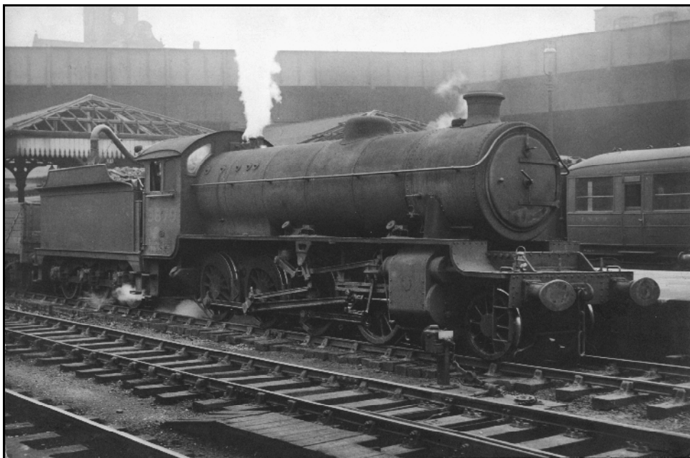
LNOR class O1 2-8-0 no.3879 pauses to take water at Nottingham Victoria while working a down goods. Rebuilt from O4/2 no.6288 in Nov. 1944 and received new LNER number in June 1946. Became 63879 in Jan. 1949. Was allocated to Annesley in the 1950s before moving to March and finally to Staveley where it was in the last batch of class O1s to be withdrawn in July 1965.
