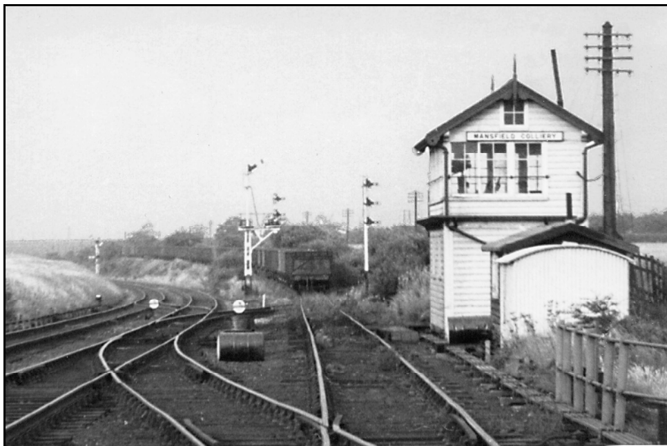
Mansfield Colliery signal box viewed looking towards Clipstone. The line to the colliery climbs up on an embankment as the colliery itself is at a higher elevation than the railway. No 34 signal is off for a train heading towards Mansfield Central.
