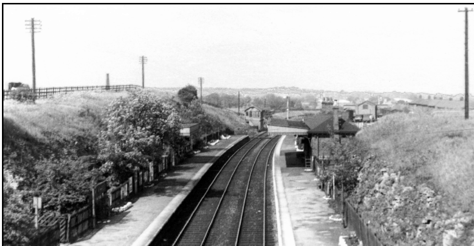
Sutton-in-Ashfield Central station looking north. The main station buildings are on the up platform and the goods shed can be seen beyond them. The signal box can be seen on the down side. photo: Douglas Thompson/Chris Booth Collection
