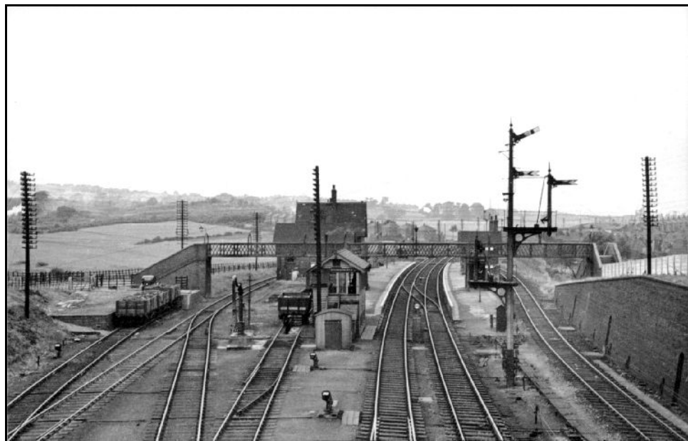
Woodhouse station in the early 1950s looking west towards Sheffield from Furnace Lane bridge. The original station only had the two platform lines with quadrupling taking place in 1912. The small goods yard on the left was accessed from the down slow line. The signal box at the platform end is Woodhouse West Junction.
